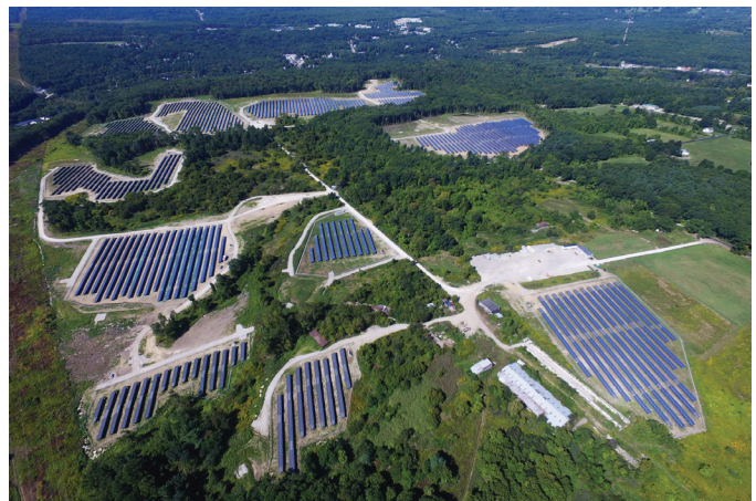
Figure 1. Utility-scale solar facilities are large-scale uses that can have significant land-use impacts on communities. Photo by Flickr user U.S. Department of Energy/Michael Faria.
