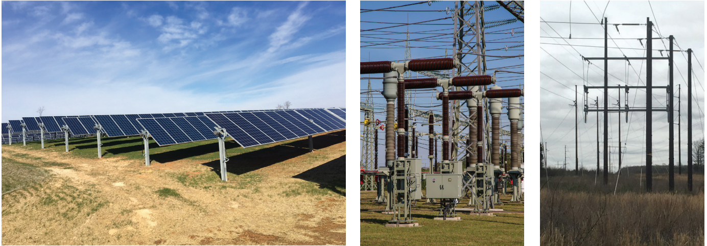
Figure 2. Components of a solar farm: solar panels (left), substation (center), and high-voltage transmission lines (right). Photos courtesy Berkley Group (left, right) and Pixabay (center).
